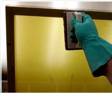
Step 1. Apply X-Bond directly to the adhesive. X-Bond will break the adhesive bond in 1-3 minutes*
